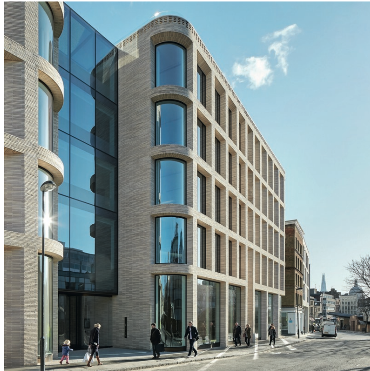
Turnmill building, London. Photo: Hufton & Crow
