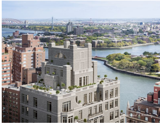
20 East End Avenue
