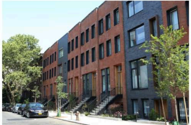
The rowhouses on State Street in Boerum Hill are credited for starting the wave of new townhouse building. Chester Higgins Jr./The New York Times
