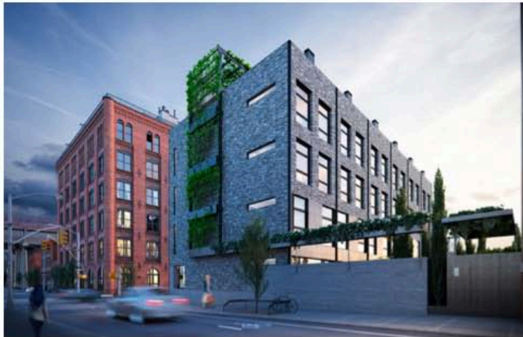
Wythe Lane Townhouses on Wythe Avenue and South Fourth Street in Williamsburg. Noë & Associates
