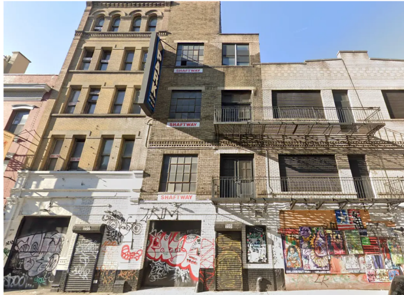
The former parking garage at 220 East 9th Street. Streetview © 2024 Google
